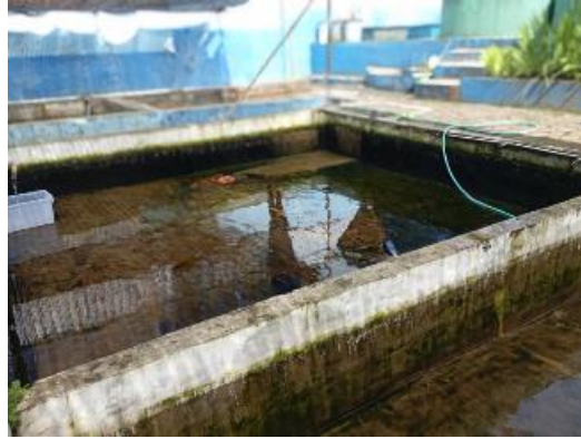
Figure 2: Concrete pool preparation
